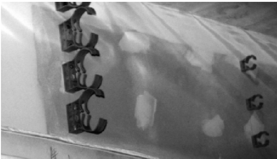
CLIC supports installed for piping to accept bare and insulated tubing
