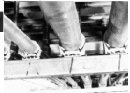
(Above left) Assembled trapezes allows less onsite parts and labor.
