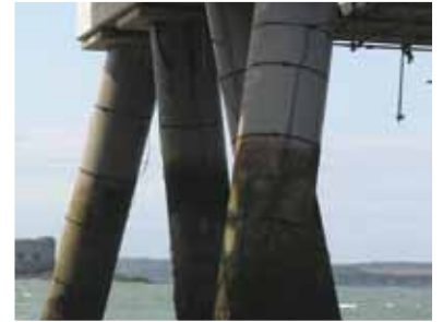
Corrosion Protection - Anode Attachment
