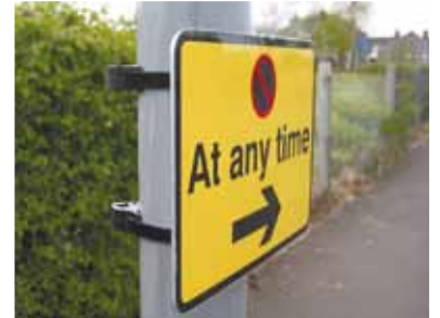
Street Furniture - Sign Fixing
