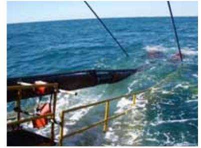
Piggyback Clamp Pipelay
