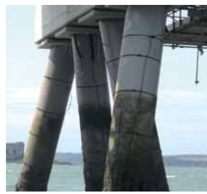
Milford Haven Cathodic Protection Project Client: Corrosion Control Services Ltd
